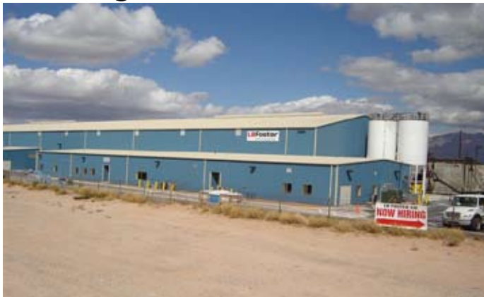
LB Foster - CXT manufacturing facility in Tucson, Arizona by Fast Fab Erectors, Inc.
